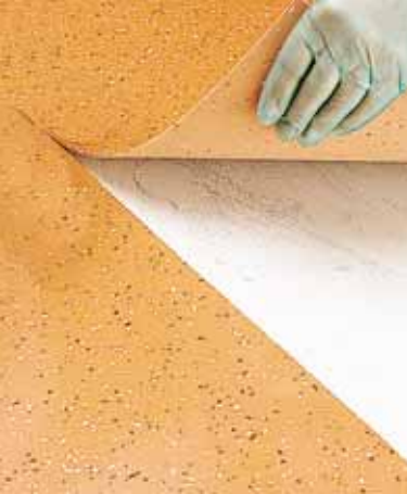
Installation of PVC with Adesilex G20
